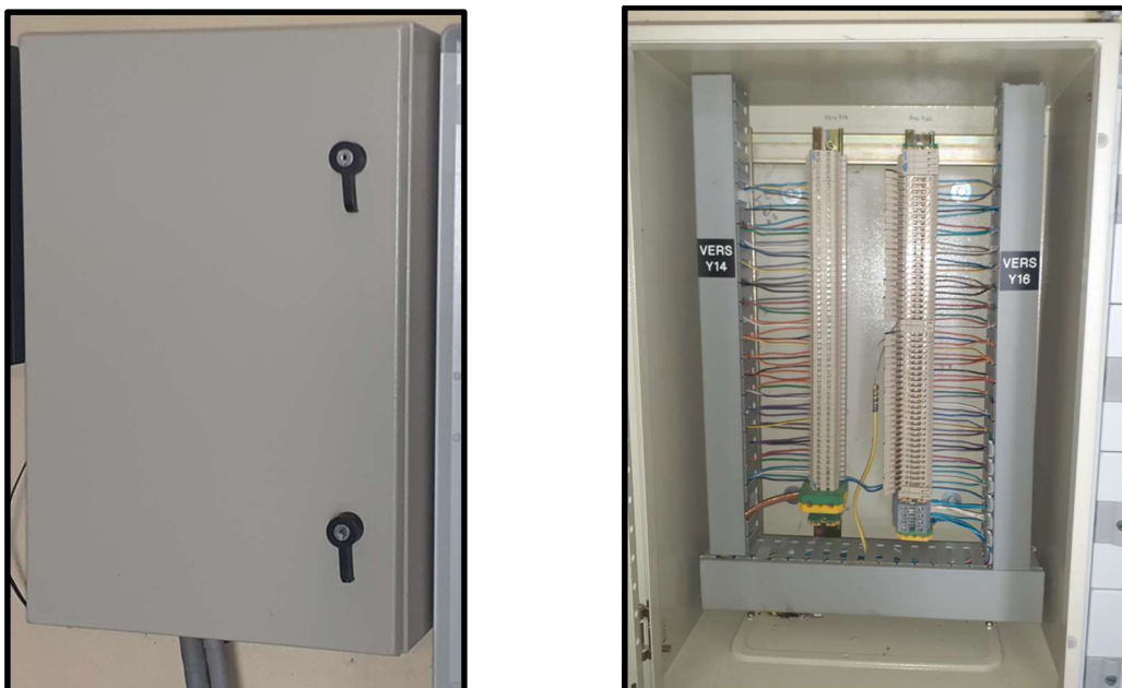
Coffret bornier de transmission
